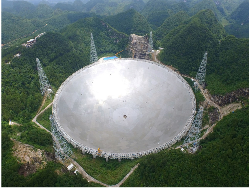
Figure 3. FAST Radio Telescope (500 m cable-suspended robot) in China
